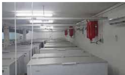
Automatic fire suppression system capable of alerting and extinguishing fire within seconds after it starts is installed in the regional genebank
