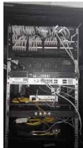
Newly installed rack for servers, UPS and cable terminals
