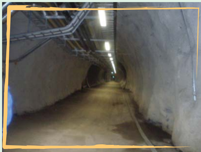
A tube leading to the chambers
